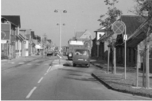
Figure 2.2. Danish Environmentally Adapted Through Road. (Vinderup, Denmark)
