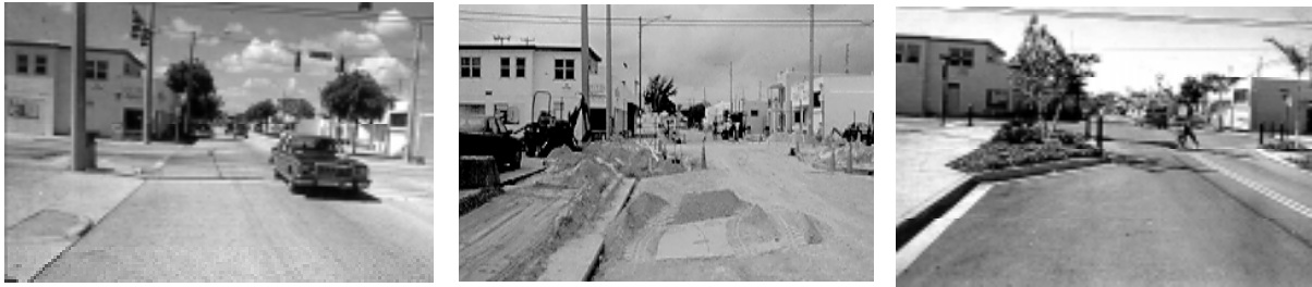
Figure 1.8. Before, During, and After Commercial Area Revitalization. (West Palm Beach, FL)
